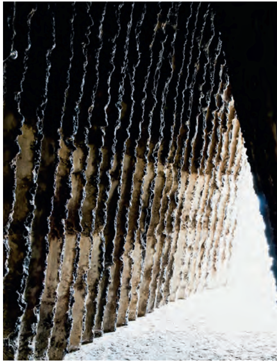
Fig. 7.6 Bruder Klaus Field Chapel: Traces of burned trunks used to cast the reinforced concrete walls
