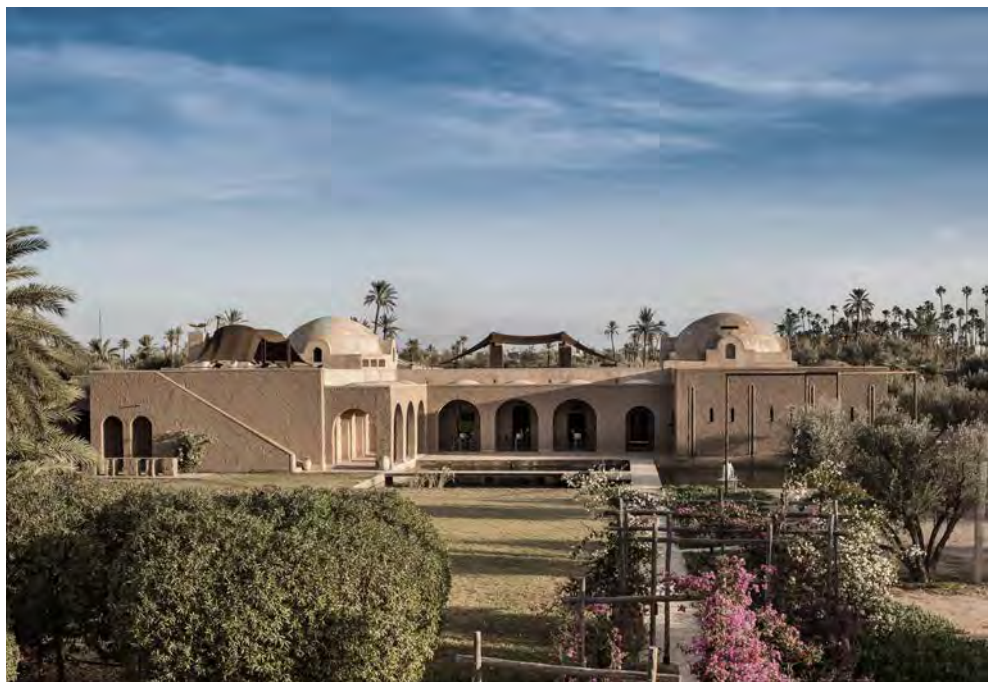
Centre Villa Janna, Marakech (Maroc), 2016, arch. Denis Coquard
