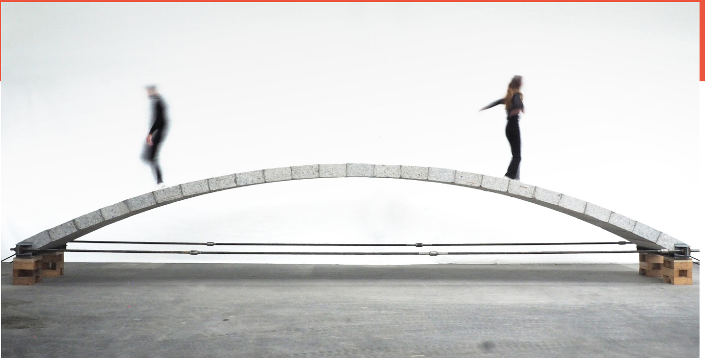
Footbridge using reinforced-concrete blocks from walls of a building being renovated
